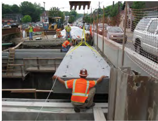
Placing a Hybrid Composite Beam
