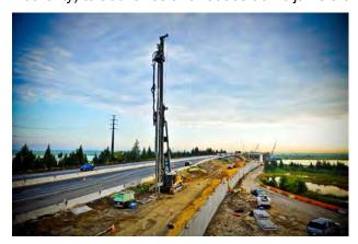
The specifications called for construction of a two-stage Mechanically Stabilized Earth (MSE) wall with stone columns and a waiting period. This process can be both expensive and time consuming. Bridgeville-based ground improvement contractor Menard teamed with its sister company. MSE wall supplier designer Reinforced Earth Company (RECo), to provide a value engineered solution. The two proposed a one-stage MSE wall system on Controlled Modulus Columns (CMC. This design allowed for
